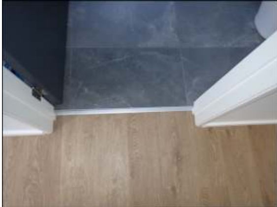
Floor material change from timber flooring to tile in bathroom appeared in good condition. No crack or damage noticed.
