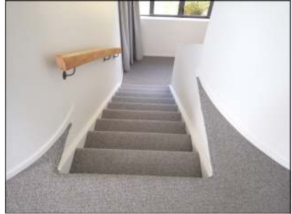
Stairs on carpet floor secured with timber handrail appeared in good condition without damage or buckling noticed. No evidence of leaky condition noticed.
