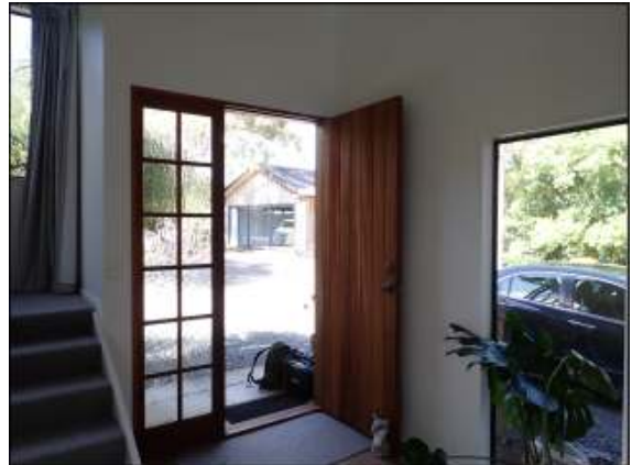
Foyer area on timber flooring appeared in good condition without damage or buckling noticed. No evidence of leaky condition noticed.
