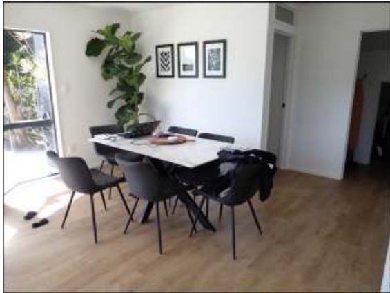
Dining area on timber flooring appeared in good condition without damage or buckling noticed. No evidence of leaky condition noticed.
