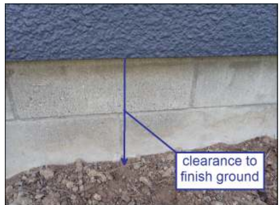
Bottom of of EIFS exterior wall cladding cleared to finish ground appeared in good condition without damage or anomaly noticed.
