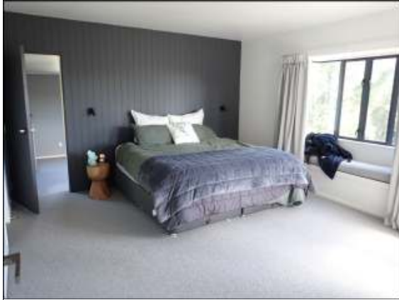
Master bedroom on carpet floor appeared in good condition. No damage or buckling noticed. No evidence of leaky condition noticed.
