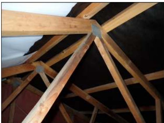
Roofing paper secured on timber roof frame without trace of leaky evidence noticed.
