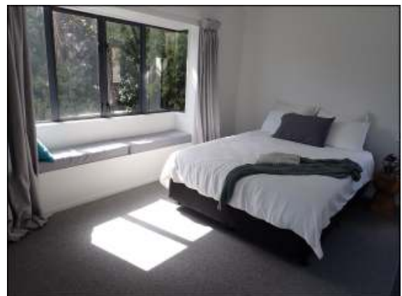
Bedroom IV on carpet floor appeared in good condition. No damage or buckling noticed. No evidence of leaky condition noticed.
