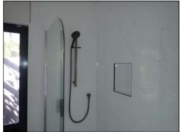
Built-in on wall shower appeared in good condition. No damage or anomaly noticed.
