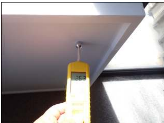
Photo 30.5 Normal level of moisture detected on wall facing exterior in master bedroom. Optimal level shall be between 20 and 40.
