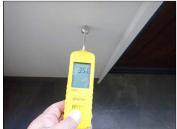
Photo 28.4 Normal level of moisture detected on wall facing exterior in bedroom II. Optimal level shall be between 20 and 40.
