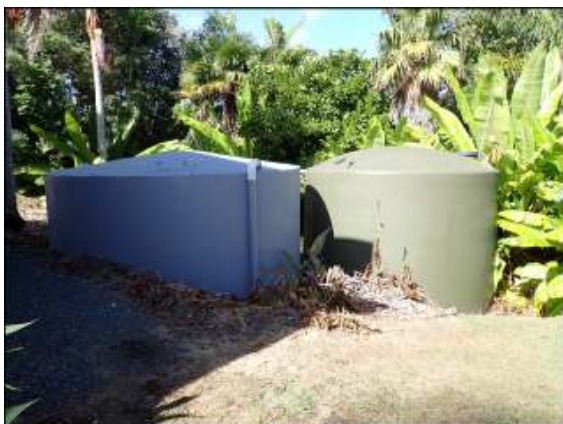
Rain water collecting tank secured on ground appeared in good condition. No damage or anomaly noticed
