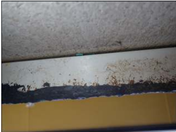
Under side of EIFS(Exterior Insulation & Finish System) exterior wall cladding appeared in good condition without damage or anomaly noticed.
