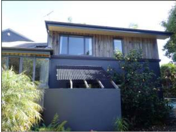
South facade with metal joinery on exterior wall cladding appeared in good condition without damage or anomaly noticed.
