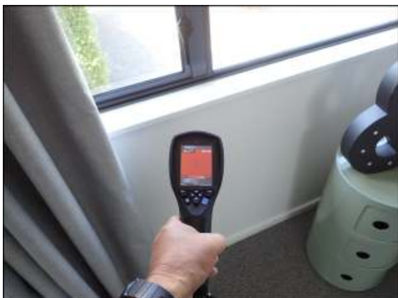
Photo 26.5 Normal level of moisture reading detected with infrared thermal imaging camera on wall facing exterior in bedroom III.
