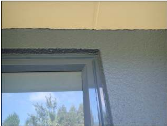
Metal joinery secured under eave appeared in good condition without damage or anomaly noticed.
