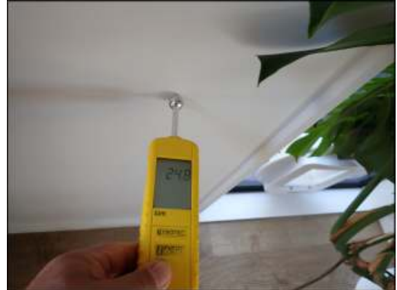
Photo 28.2 Normal level of moisture detected on wall facing exterior at foyer area. Optimal level shall be between 20 and 40.
