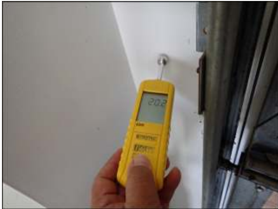
Photo 29.3 Normal level of moisture detected on wall facing exterior in garage. Optimal level shall be between 20 and 40.
