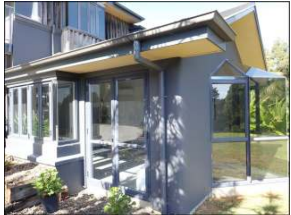
North East facade with metal joinery on exterior wall cladding appeared in good condition without damage or anomaly noticed.
