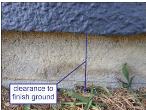
Bottom of of EIFS(Exterior Insulation & Finish System) exterior wall cladding cleared to finish ground appeared in good condition without damage or anomaly noticed.
