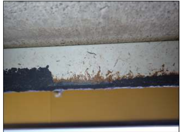
Under side of EIFS exterior wall cladding appeared in good condition without damage or anomaly noticed.
