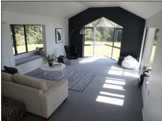
Living room on carpet floor appeared in good condition without damage or buckling noticed. No evidence of leaky condition noticed.
