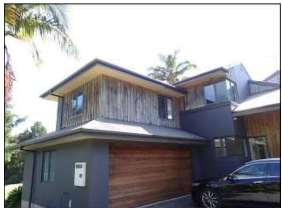
Metal joinery secured on exterior wall cladding appeared in good condition without damage or anomaly noticed.
