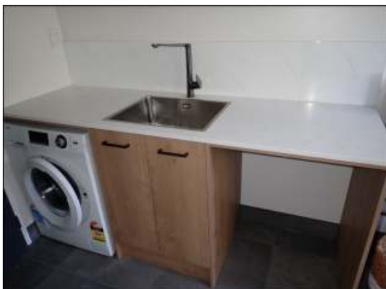
Laundry area appeared in good condition. Normal level of moisture detected on wall around laundry area.
