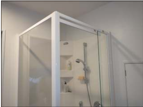
Prefabricated shower stall appeared in good condition without damage and anomaly noticed.
