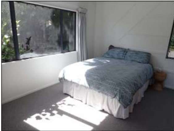
Bedroom II on carpet floor appeared in good condition. No damage or buckling noticed. No evidence of leaky condition noticed.
