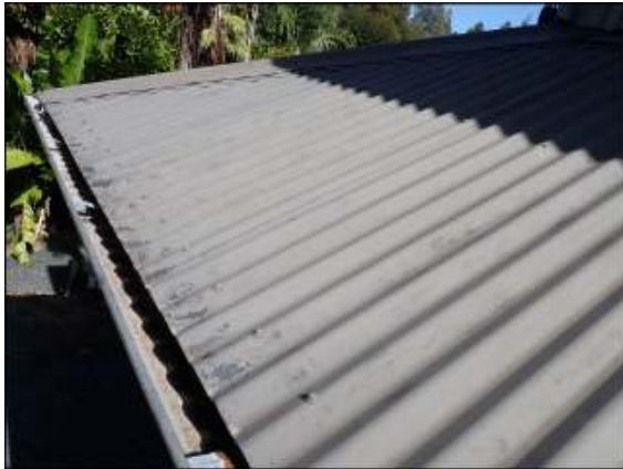
Maintained corrugated sheet metal roof appeared in good condition. No dent and/or damage noticed.
