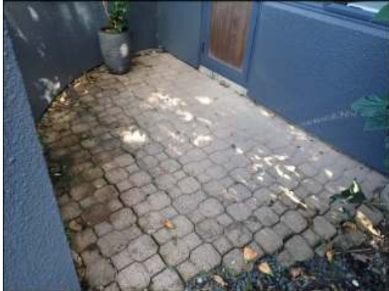
Landscape stone pavement porch appeared in good condition without crack or damage noticed.
