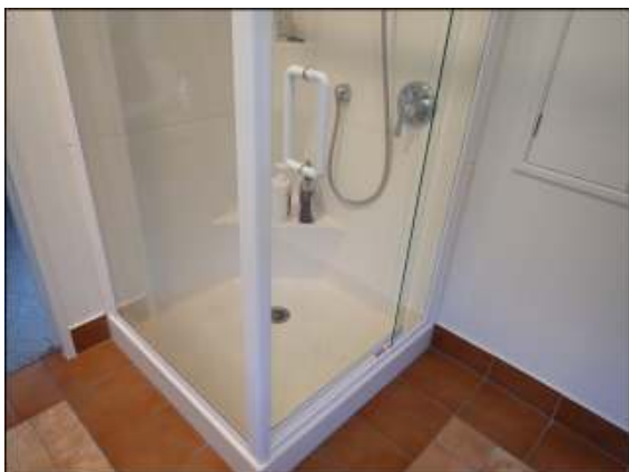
Prefabricated shower stall appeared in good condition. Normal level of moisture detected around stall.
