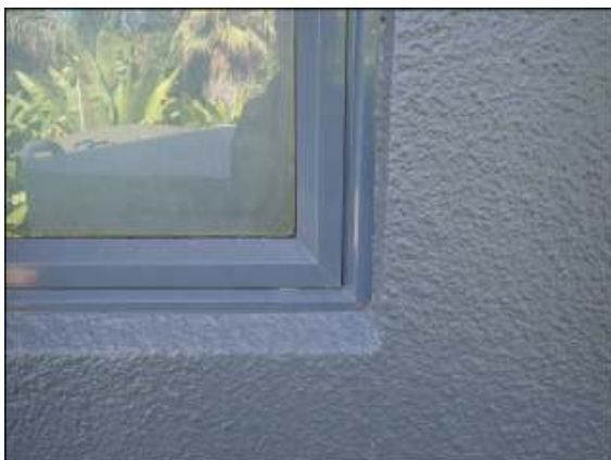
Metal joinery secured on sloped sill on exterior wall cladding appeared in good condition without damage or anomaly noticed.
