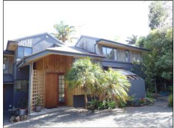
South main facade with metal joinery on exterior wall cladding appeared in good condition without damage noticed.
