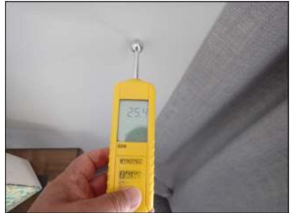
Photo 30.4 Normal level of moisture detected on wall facing exterior in family room. Optimal level shall be between 20 and 40.
