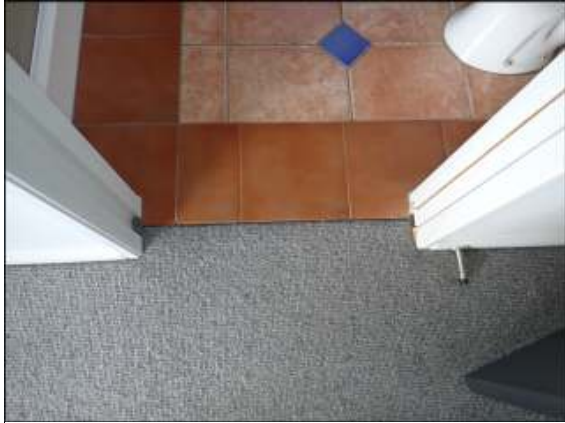
Floor material change from carpet to tile at en suite bathroom appeared in good condition. No crack or damage noticed.
