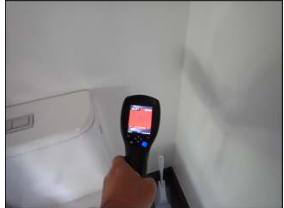
Normal level of moisture reading with infrared thermal imaging camera on wall around toilet.
