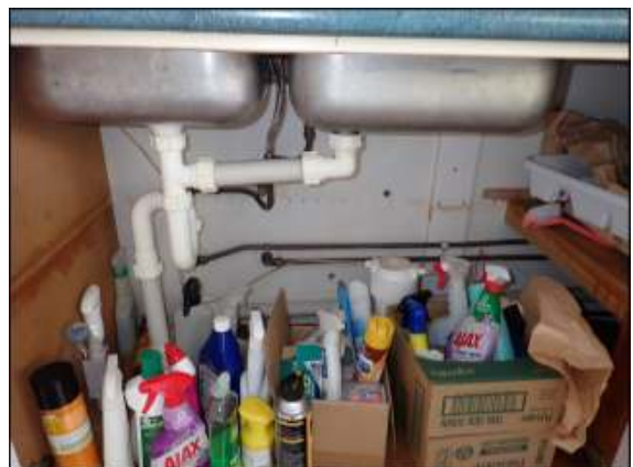
U-trap without garbage dispense appeared in good condition without damage noticed.
