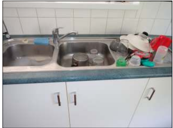
Stainless steel sink secured on work bench appeared in good condition.
