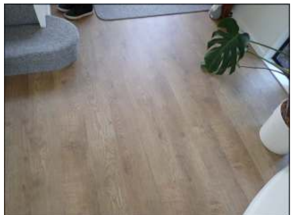
Hallway on timber flooring appeared in good condition without damage or buckling noticed.
