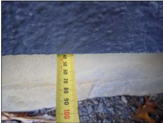
Bottom of of EIFS exterior wall cladding appeared in good condition without damage or anomaly noticed.
