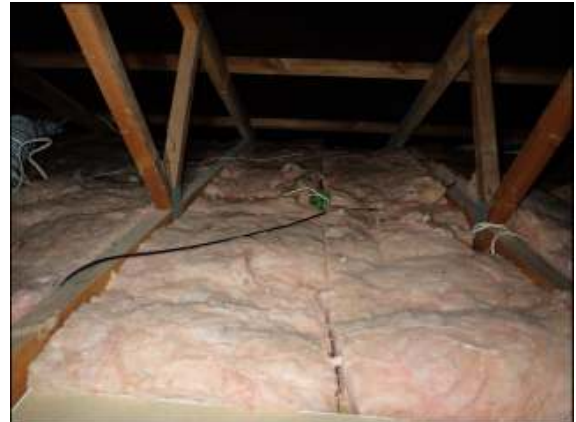
Roofing paper secured on timber roof frame. Fibreglass blanket insulation laid in with R-1.8 approximately.
