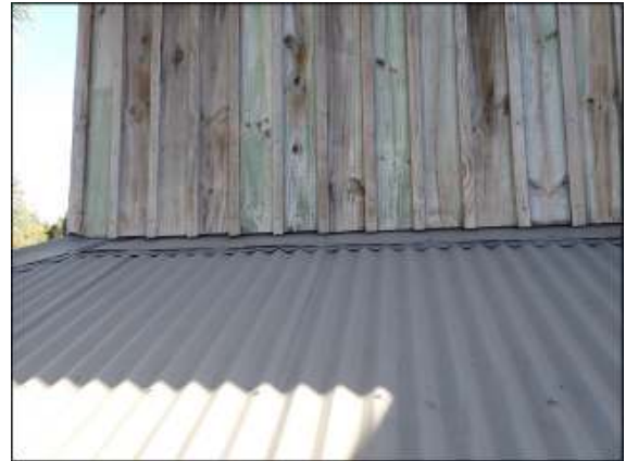
Exterior wall cladding cleared to finish roof, secured with metal flashing, appeared in good condition without damage or anomaly noticed.
