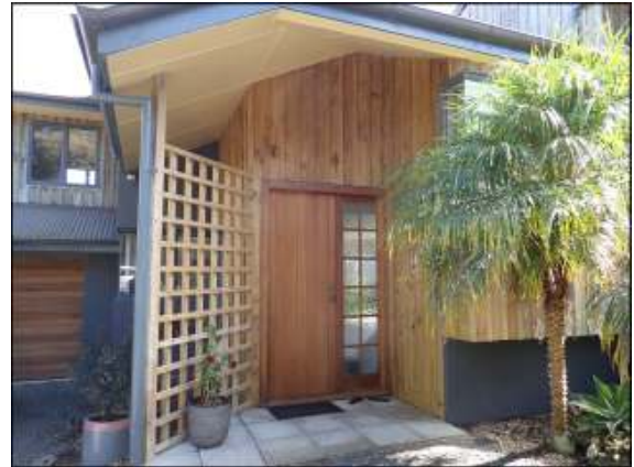
Main entrance door secured under covered walkway appeared in good condition.
