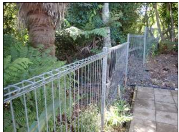
Metal fence appeared in good condition without damage or sign of out of verticality noticed.
