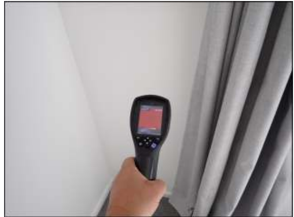
Photo 25.4 Normal level of moisture reading detected with infrared thermal imaging camera on wall facing exterior in bedroom II.
