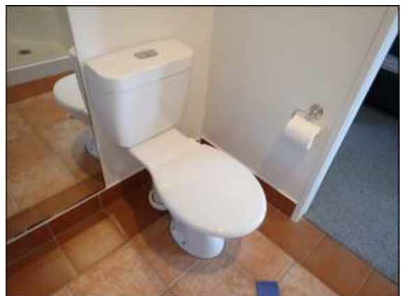
Ceramic toilet secured on floor without damage or dislocation was noticed. Normal level of moisture detected around toilet.
