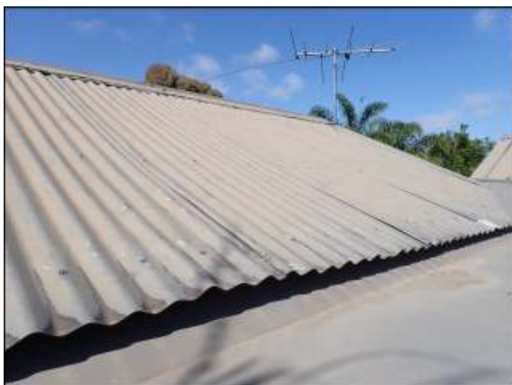
Corrugated sheet metal roof appeared in good condition at valley without damage noticed.
