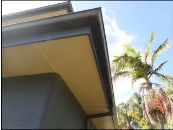
Metal gutter secured on barge board appeared in good condition without damage. Noticed internal guttering system installed.
