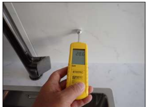
Normal level of moisture detected on wall around laundry connection. Optimal level shall be between 20 and 40.
