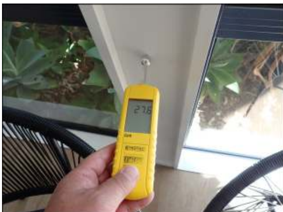
Photo 28.5 Normal level of moisture detected on wall facing exterior at kitchen/dining area. Optimal level shall be between 20 and 40.
