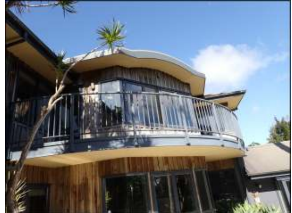
Cantilever balcony secured with guardrail appeared in good condition without damage or anomaly noticed.
