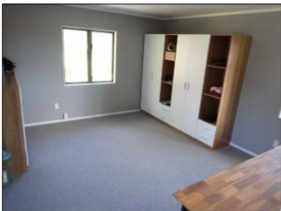
Studio at mezzanine on carpet floor appeared in good condition without damage or buckling. No evidence of leaky condition noticed.
