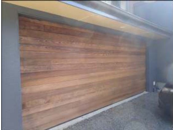
Timber overhead panel garage door outside appeared in good condition.
