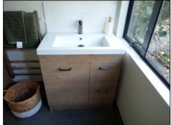
Hand wash basin and vanity appeared in good condition without crack or damage.
