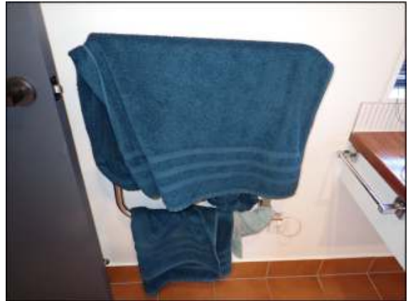
Electric towel dry hanger secured on wall. Operation was tested and working OK.
