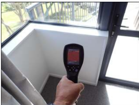
Photo 27.5 Normal level of moisture reading detected with infrared thermal imaging camera on wall facing exterior in master bedroom.
