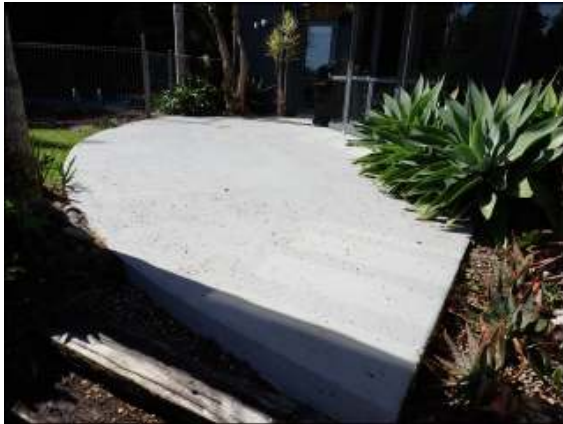
Concrete pavement porch appeared in good condition without crack or damage noticed.
